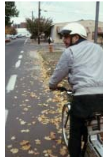
Leaf Debris on Roadway Source: Dan Burden
