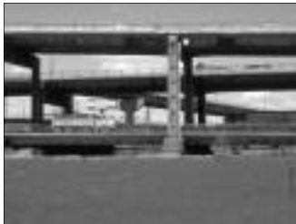
The Gardiner Expressway and Lakeshore Blvd. crossing the Don River.
